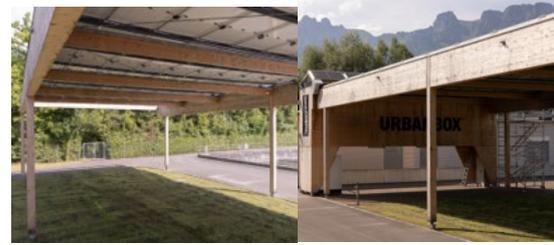
**Figure 2:** Wood is used as relevant construction material in the URBANBOX base construction.
