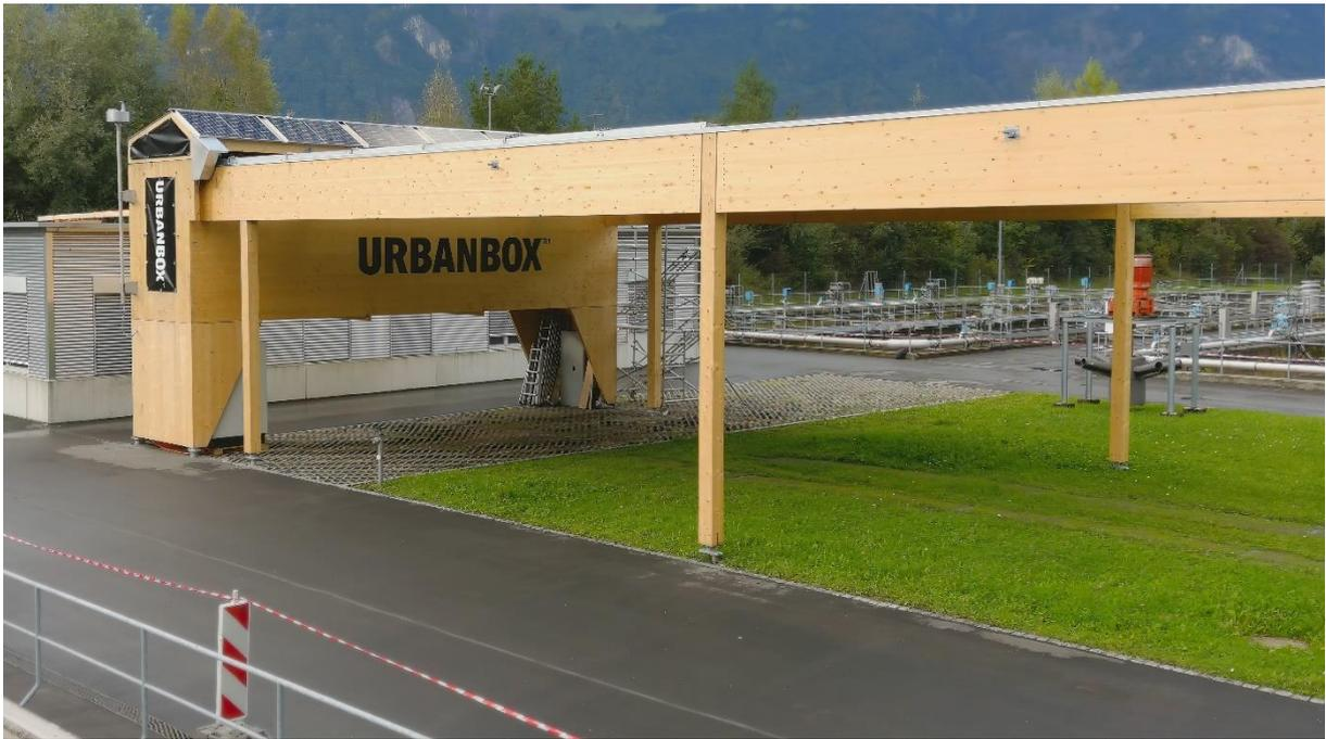
**Image 6** : Views from Urbanbox demonstration system with 6 PV module supports extended (Image: Iworks AG).
