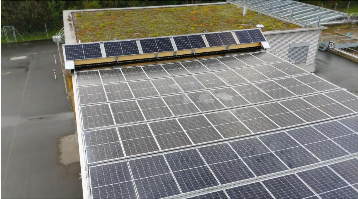
**Image 5** : Views from Urbanbox demonstration system with 6 PV module supports extended (Image: Iworks AG).
