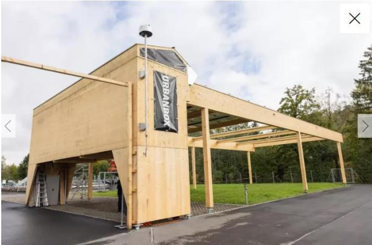
With a retractable photovoltaic roof over sewage treatment plants, parking lots or roads to produce electricity: That's the idea behind the Urbanbox. Yesterday of the lightweight photovoltaic system at the ARA wastewater treatment plant in Bendern. Photo by Daniel Schwendener
